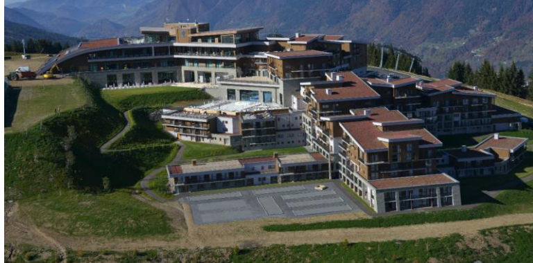
Club Med Hotel in Samoëns Architect: Studio Arch
